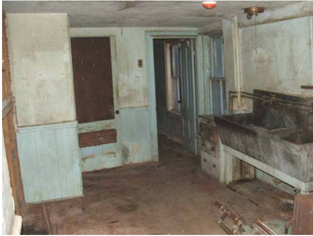
Figure 71 Kitchen c. 1900 Soapstone Sink
