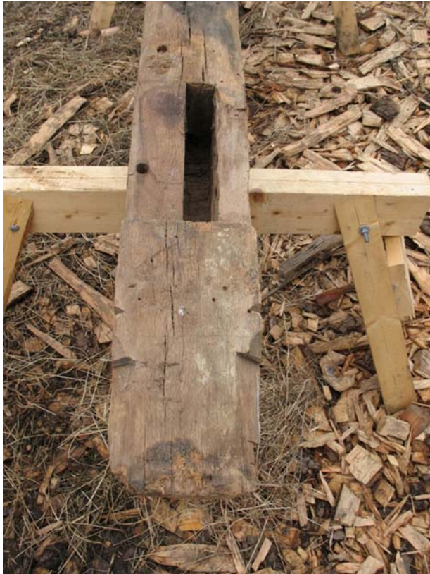
Figure 75 17thc. Re-used Post, Chamfer Detail
