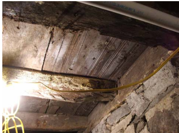
Figure 78 Barrett Muster Room floor, Basement 17thc. sheathing patch
