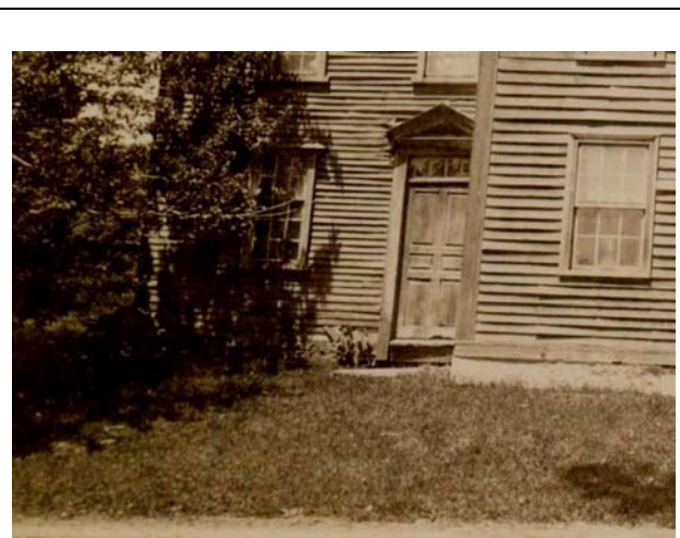
Figure 32 Barrett Ell Entry c. 1880s Detail HNE Entry had a pediment, four light bulls-eye transom and six-panel door.
