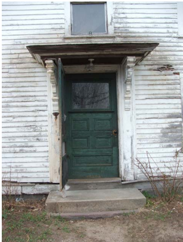
Figure 58 Barrett Front Doorway, McGrath era
