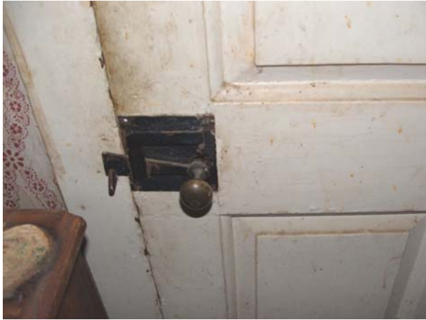
Figure 83 2nd floor E. Chamber N 18th c. door hardware
