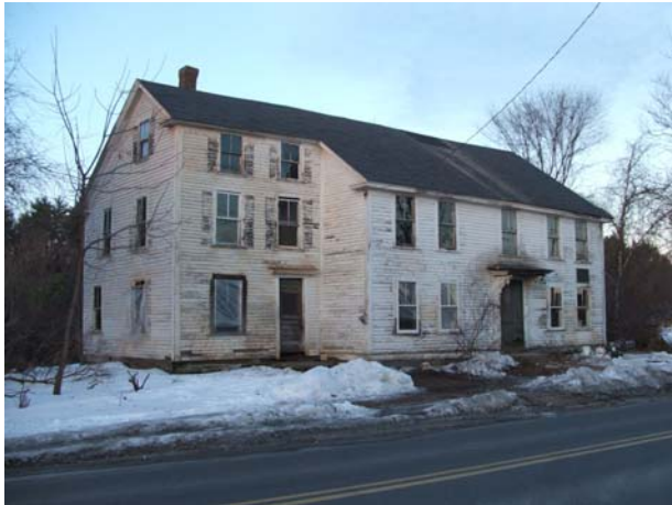
Figure 55 Col. James Barrett House SW View Dec. 2005
