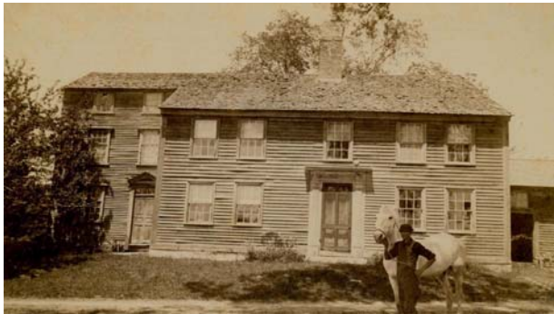
Figure 35 Barrett Farm ca.1880s with horse HNE West Ell's rived clapboards, 9/6 windows with caps, Barrett horse.
