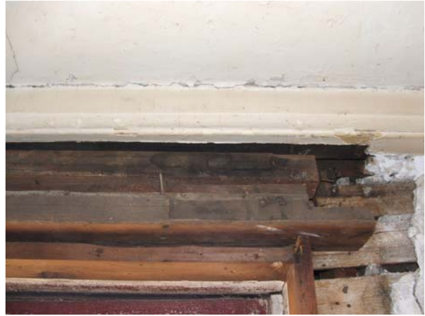
Figure 100 Barrett Muster Room 18th c. window frame fragment
