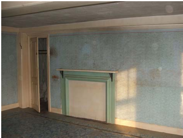
Figure 77 West Chamber 18thc. bolection on fireplace opening.view NE
