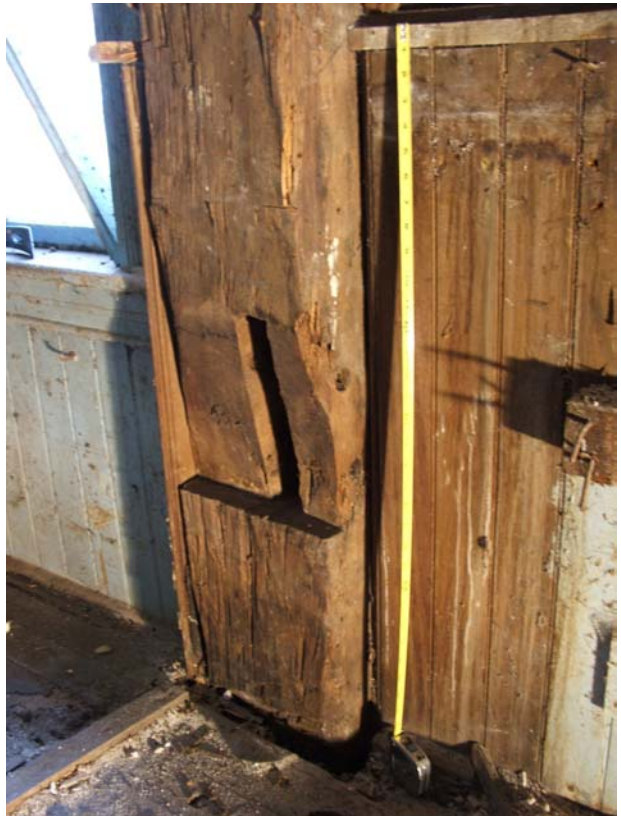
Figure 74 Kitchen re-used early chamfered post
