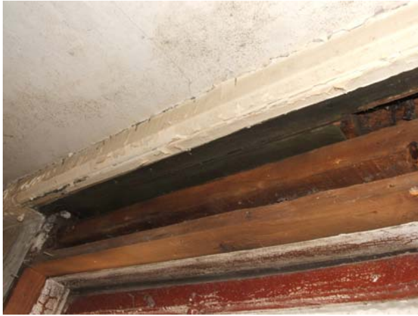
Figure 99 Muster Room 18th c. window trim evidence
