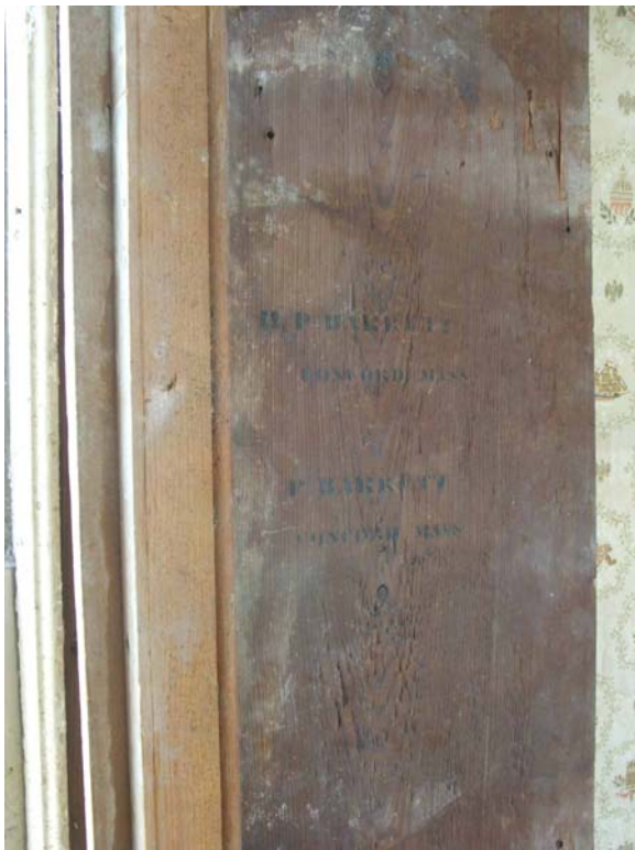
Figure 73 Second floor rear door jamb, re-used partition board
