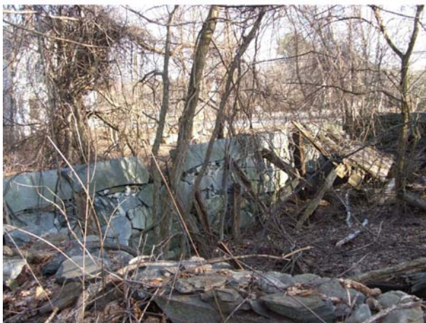
Figure 57 Barrett Barn ca. 1970 and foundation ruins 2006
