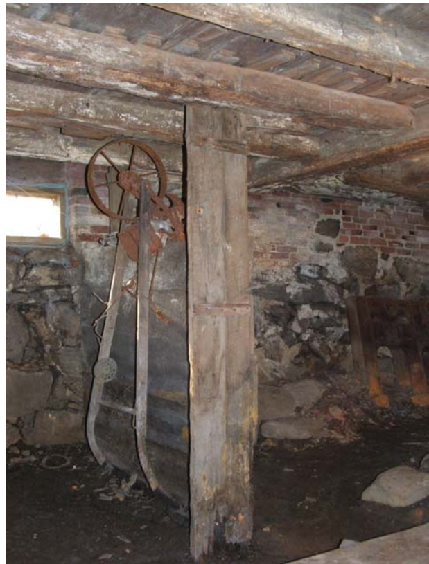
Figure 102 Barrett Muster Room Basement Artifact
