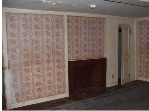
Figure 84 E. Chamber View NW. 18thc. doors, c.1800 fireplace infill
