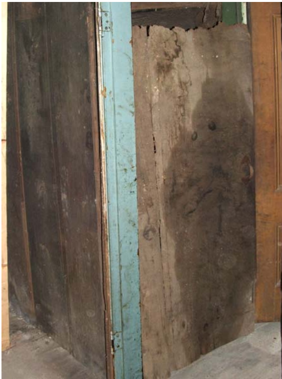
Figure 81 Kitchen / Basement Batten Door, 18thc. hw
