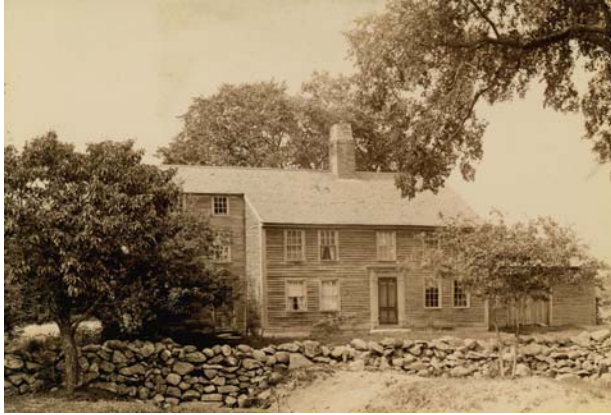
Figure 37 ca. 1880s SW View ditch, wall HNE High stone wall, deep drainage ditch, culvert lintel, fruit tree.
