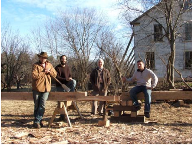
Figure 59 Barrett Repair Crew Dec. 2006
