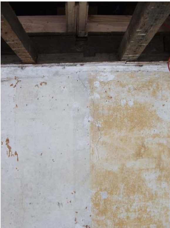
Figure 93 2nd floor former partition line, ochre whitewash
