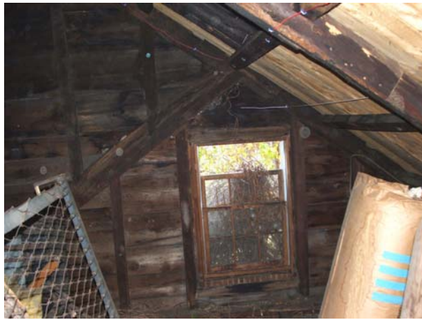
Figure 87 Barrett Attic 18thc. gable, View E
