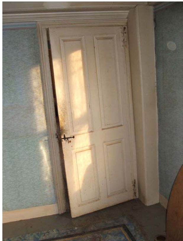
Figure 82 West Chamber SE door, 18thc. H hinges
