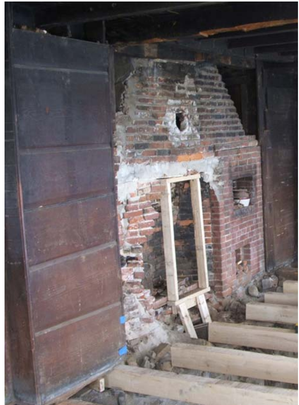
Figure 70 Kitchen Fireplace Wall, 18thc. sheathing
