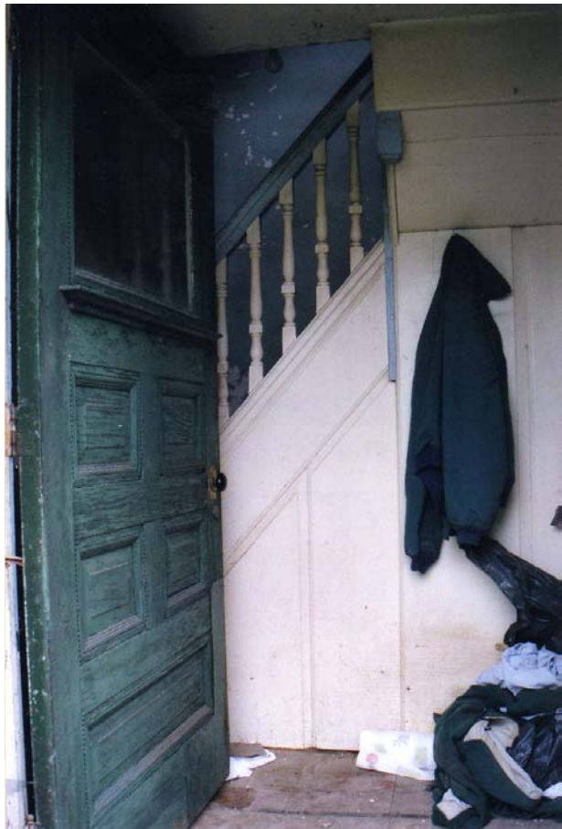
Figure 62 Barrett Entry and stairway view N
