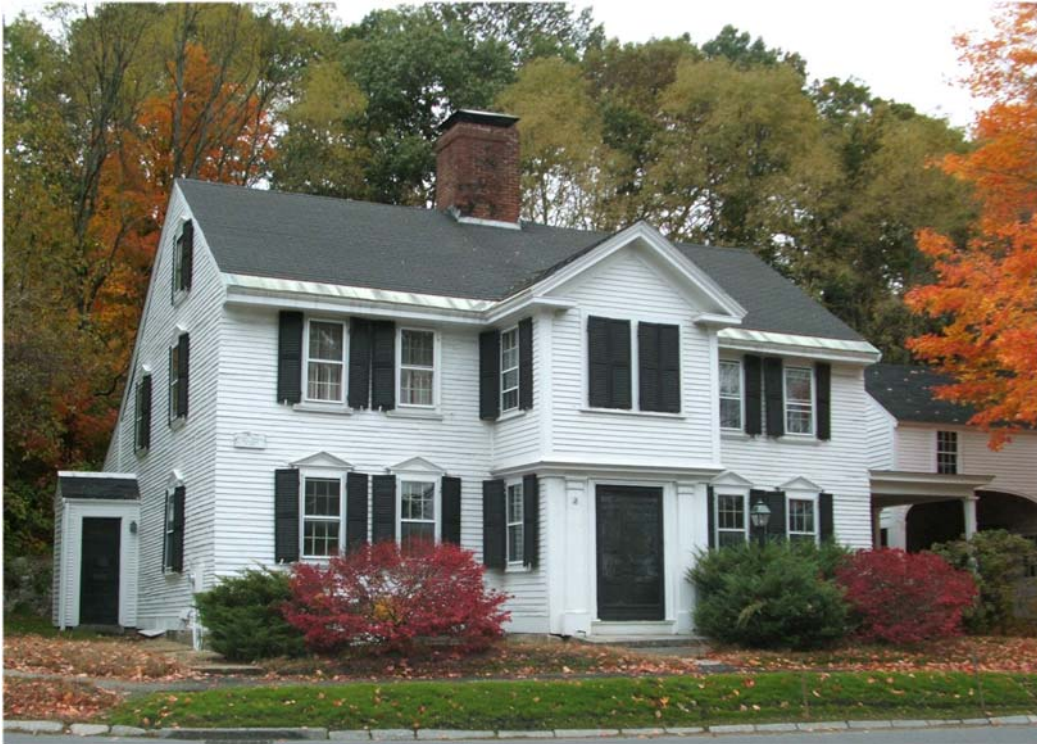
Figure 5 Beaton-Heywood House had saltbox form, window pediments The house also retains its early, skived clapboards extending to the corners.
