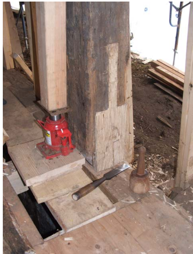
Figure 90 Kitchen Post Base Repair, 2007
