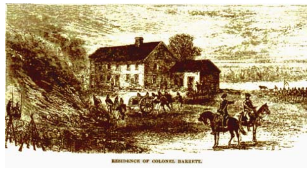
Figure 26 Barrett Farm Concord Fight Harpers 1875 A centennial view shows the east ell much as shown in later photos.
