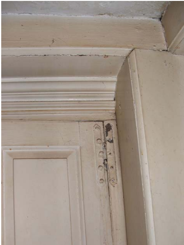
Figure 85 W Chamber Door H hinge detail
