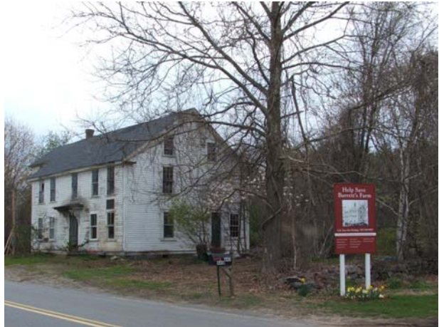
Figure 56 Col. James Barrett House SE View April 2006
