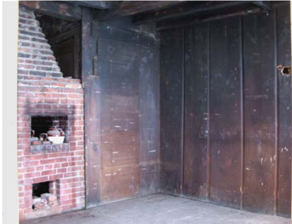
Figure 91 Barrett Kitchen SW 18th c. partition sheathing
